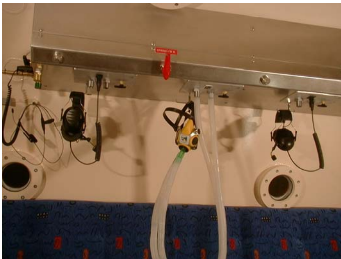
Nozzles in stainless steel mounted in a internal panel.
